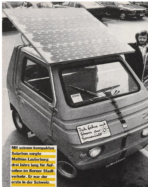
Swiss Matthias Lauterburg with his ZeleZagato with 4 Arco Solar (132 Wp) in Berne (1982)
